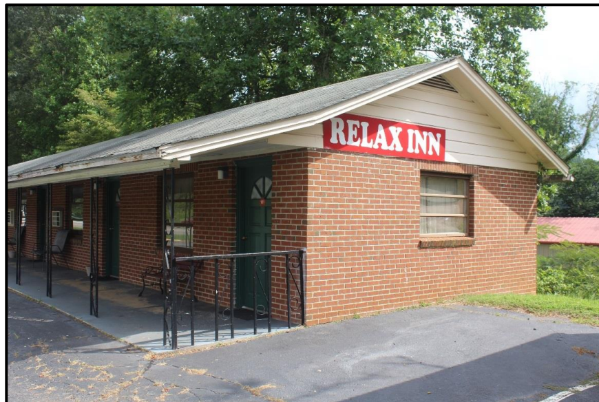
Figure 49. Detail of South Gable End of Motel, Looking Northeast.
