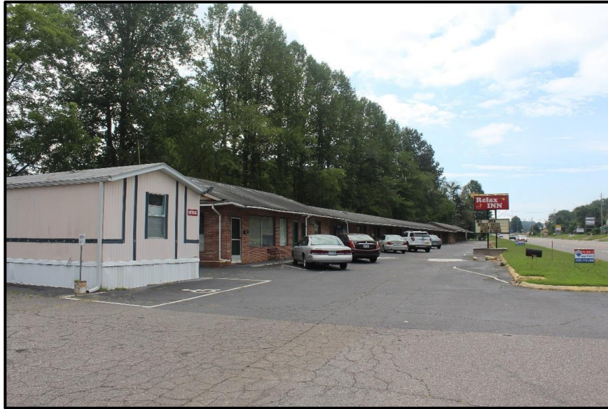
Figure 46. Relax Inn (MA0803), Looking Southeast.
