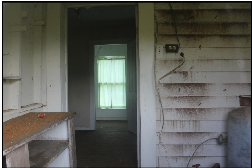
Figure 11. Interior, Looking Northwest through Window in Ell.
