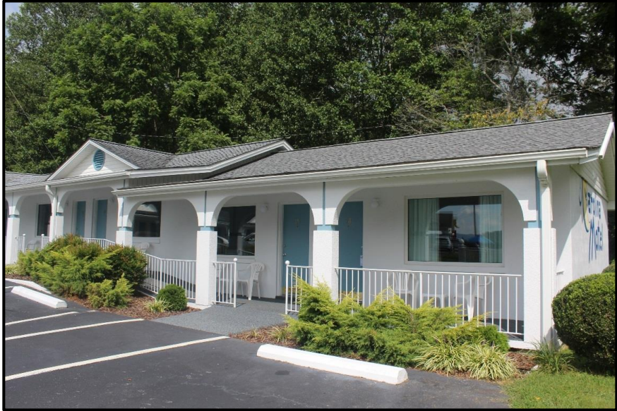
Figure 59. Eastern Section of Motel, Looking Northwest.
