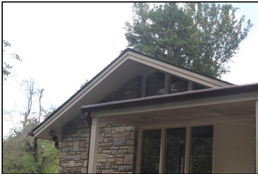
Figure 82. Detail of Gable End, Looking Southwest.
