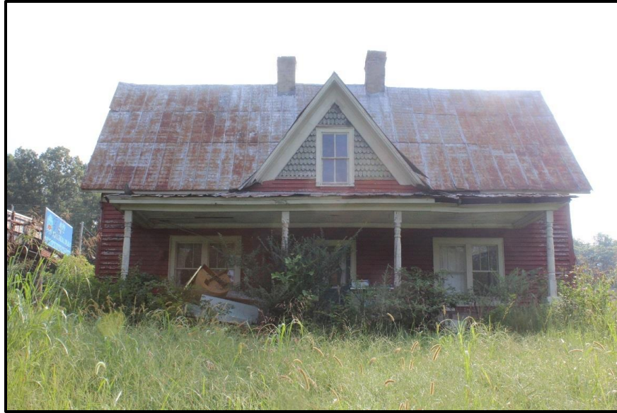
Figure 3. Union United Methodist Church Parsonage, Looking Northeast.
