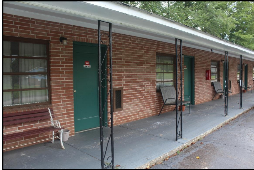
Figure 48. Detail of Porch along Front Façade of Motel, Looking Southeast.
