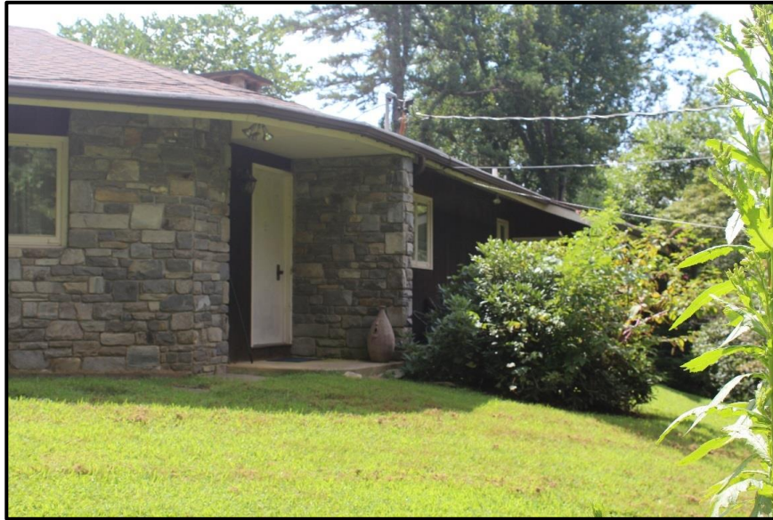
Figure 81. Detail of Front Entry, Looking Southeast.
