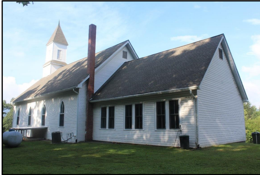
Figure 20. Union United Methodist Church (MA0305), Looking West.
