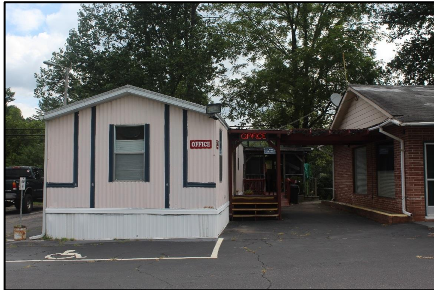
Figure 51. Motel Office, Looking East.
