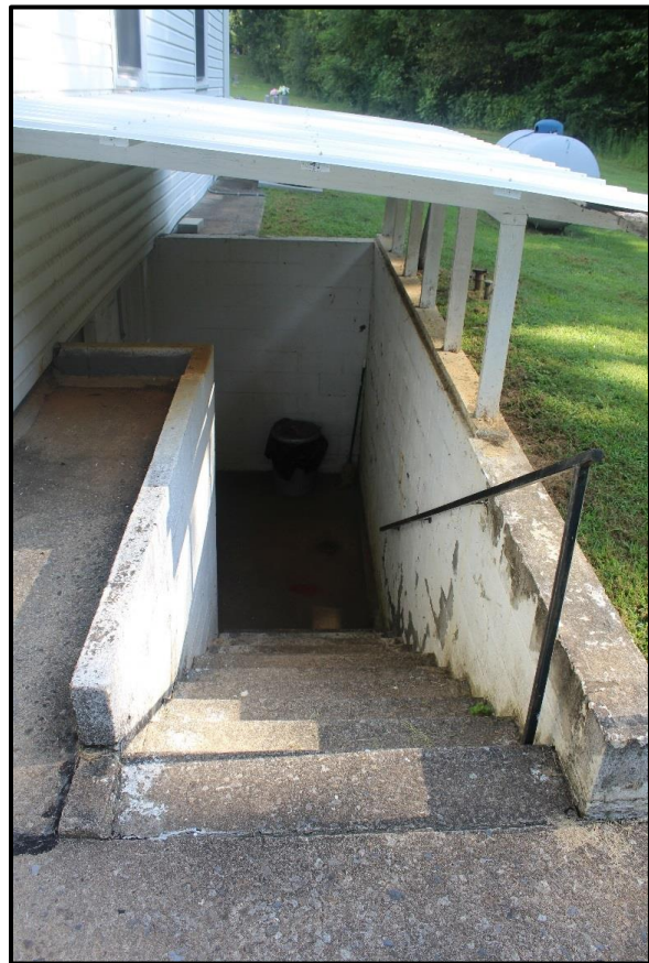
Figure 24. Stairs to Basement, Looking North.
