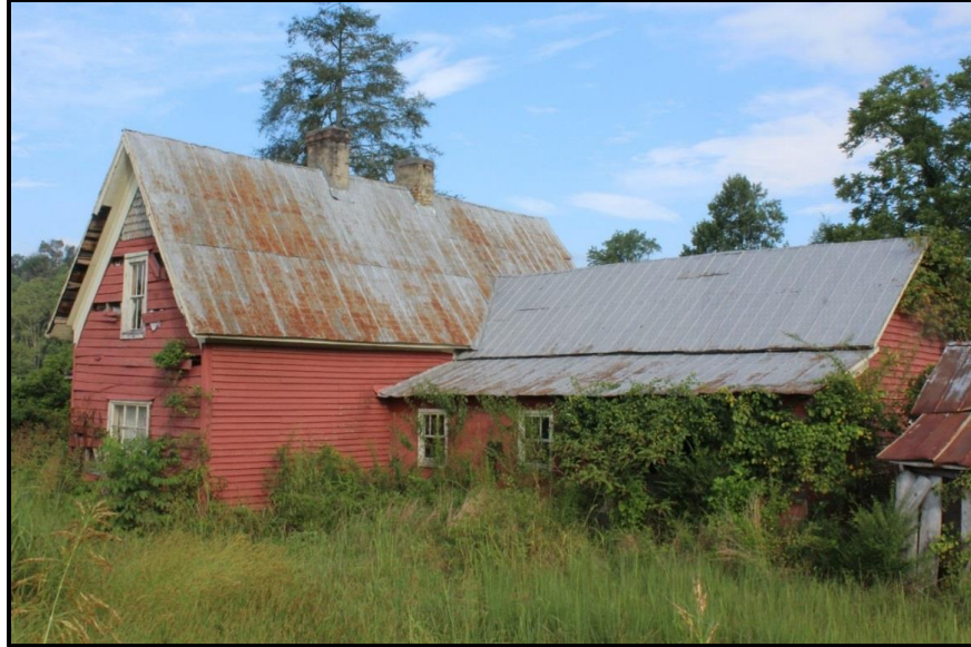
Figure 5. Union United Methodist Church Parsonage, Looking Northwest.
