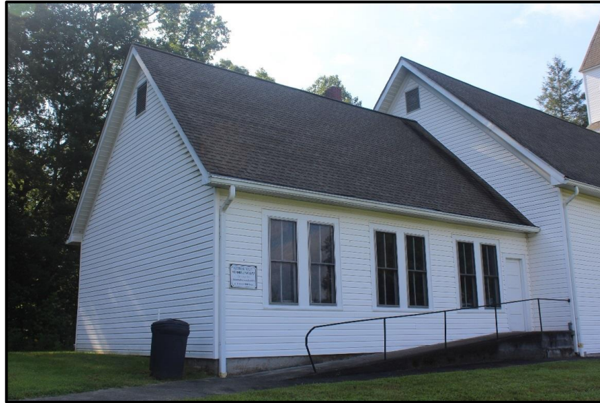
Figure 22. Rear Ell, View Looking Southeast.
