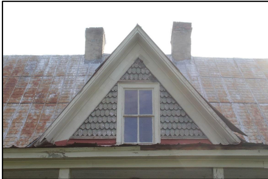
Figure 6. Detail of Projecting Pediment, Looking Northeast.
