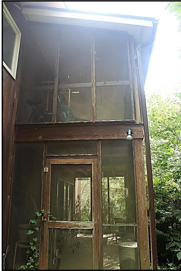
Figure 83. Porch Detail, Looking East.
