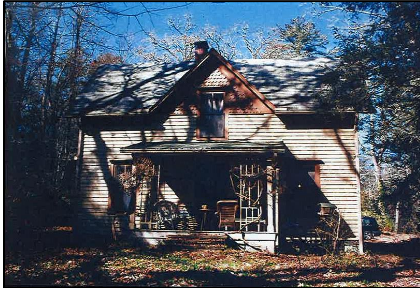
Figure 15. Edwards Family House (NRHP-Listed Highlands North Historic District), 856 North Fifth Street (Photograph from Previous Survey; HPO Site Files).
