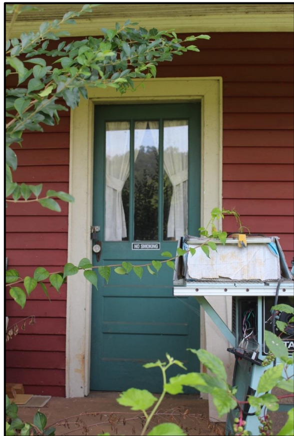
Figure 9. Entry Door, Looking Northeast.
