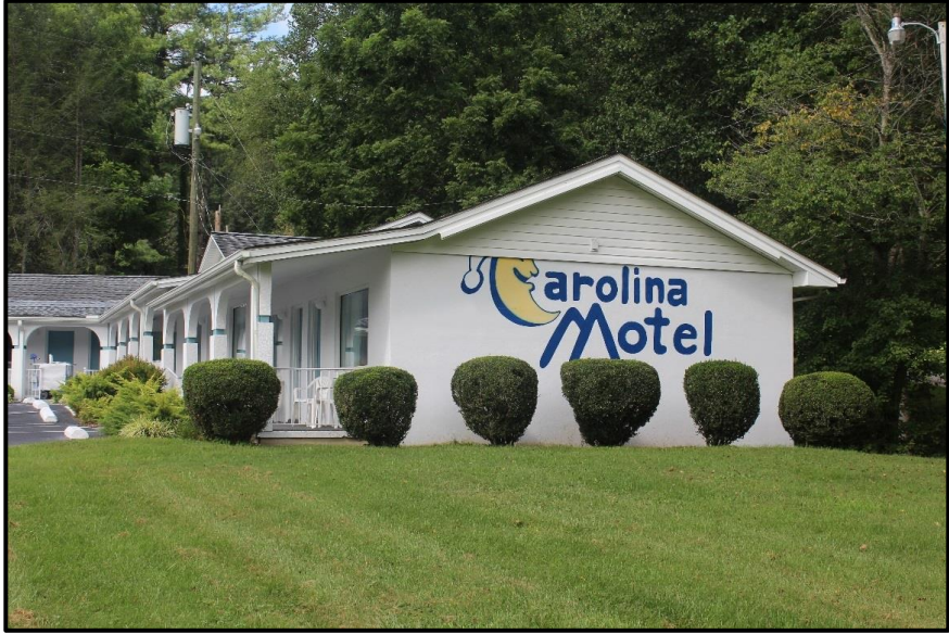
Figure 58. Detail of Eastern Gable End, Looking West.
