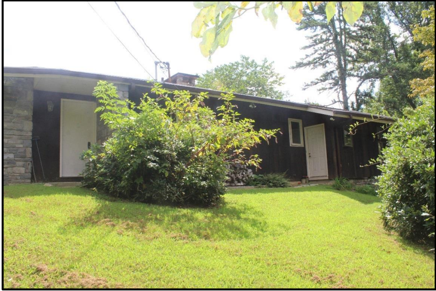
Figure 79. House, Looking Southeast.
