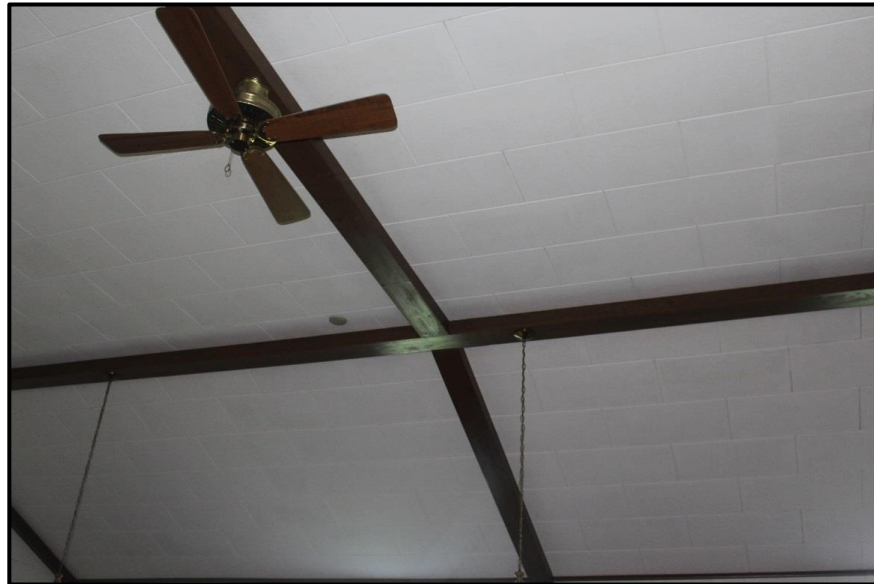
Figure 28. Detail of Ceiling.
