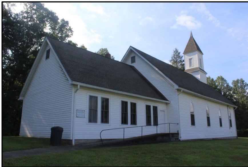
Figure 21. Union United Methodist Church (MA0305), Looking Southeast.
