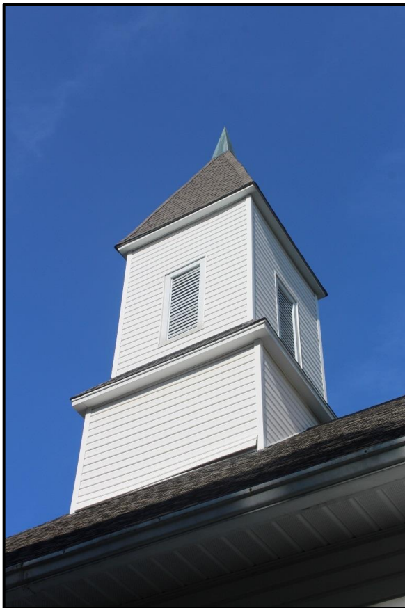
Figure 23. Detail of Bell Tower, Looking West.
