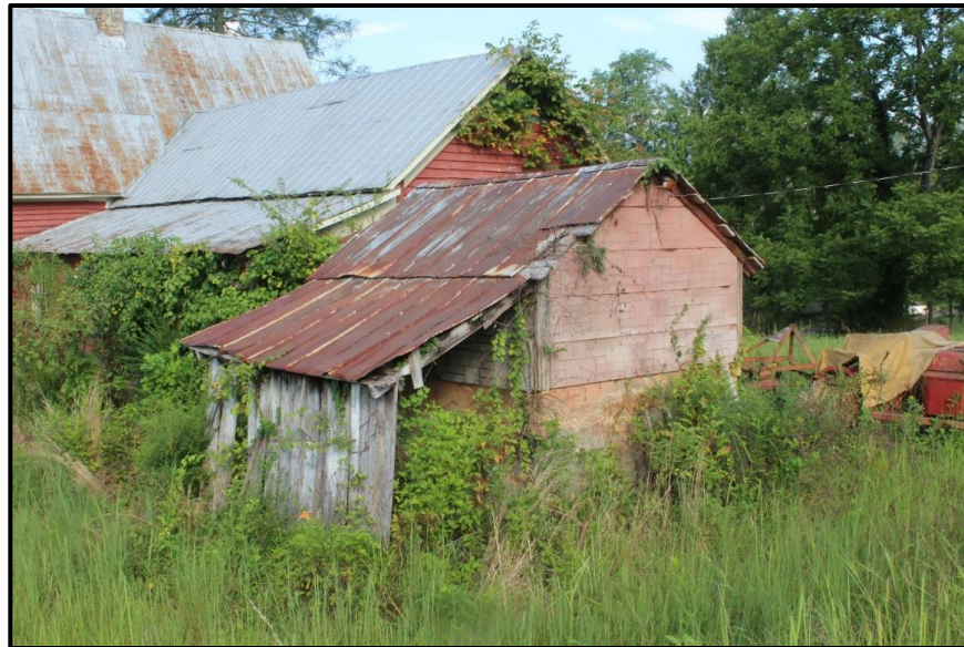
Figure 12. Canning House, Looking West.
