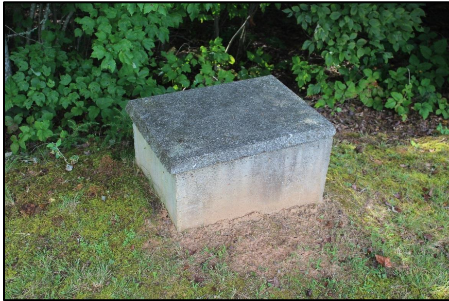
Figure 31. Poured Concrete Well, Looking Southeast.
